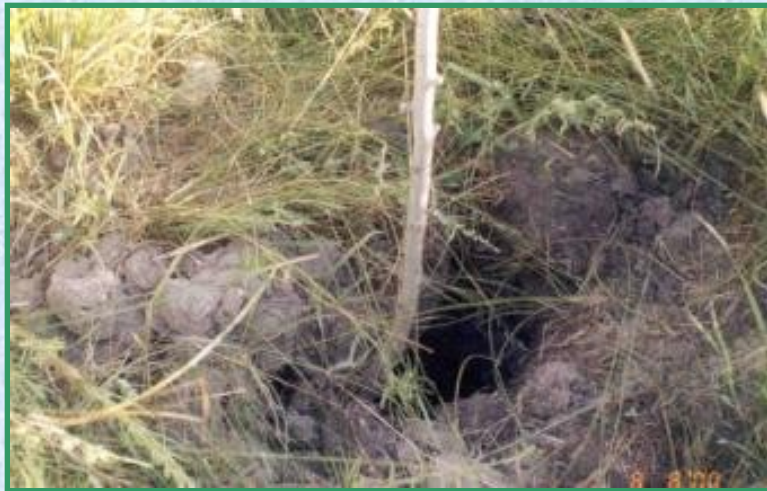
Improper backfilling
